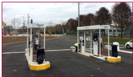
Station de gaz
