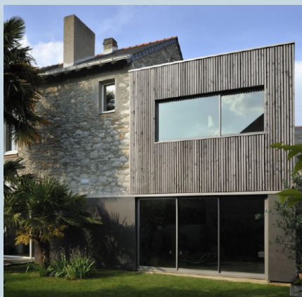
Extension bois FORMA 6 - Architecture
