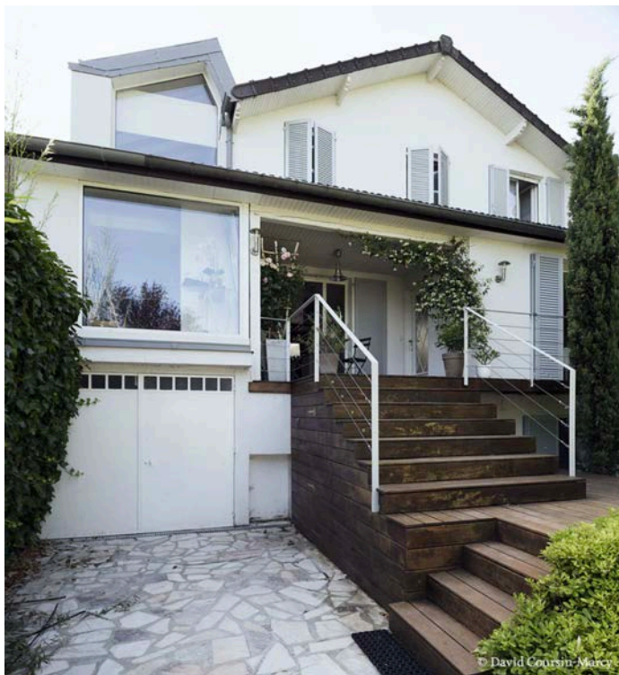
Extension maison ANGELES DUQUE - MIA ARCHITECTES
